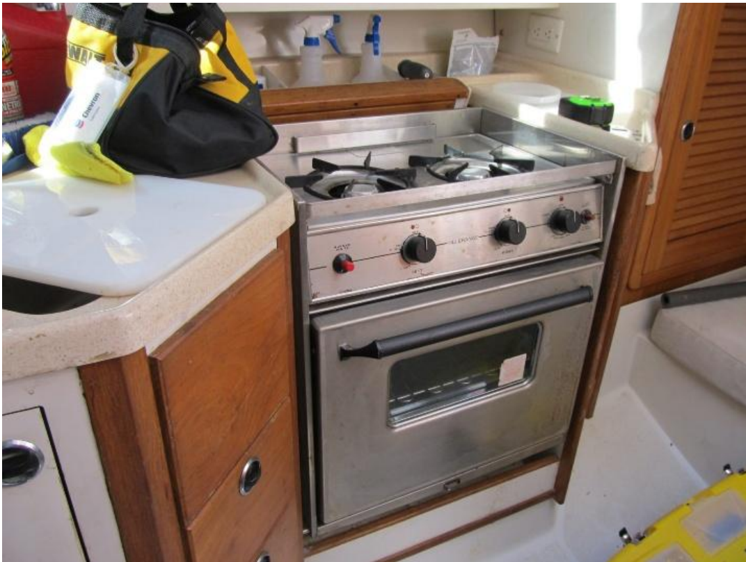
Propane, two burner stove, and oven.
