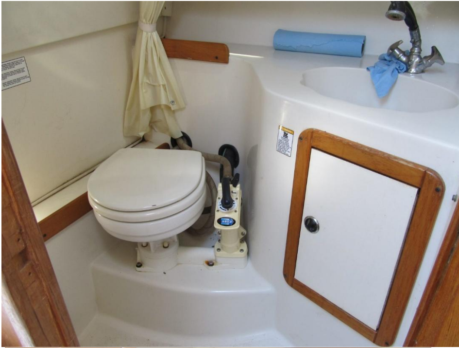
Head compartment with new head pump. "Telephone Shower" in head and on swim platform with hot water (from engine or shore power heated tank) and cold water.
