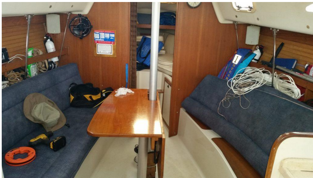
Cabin with fold out table during adding wiring.
